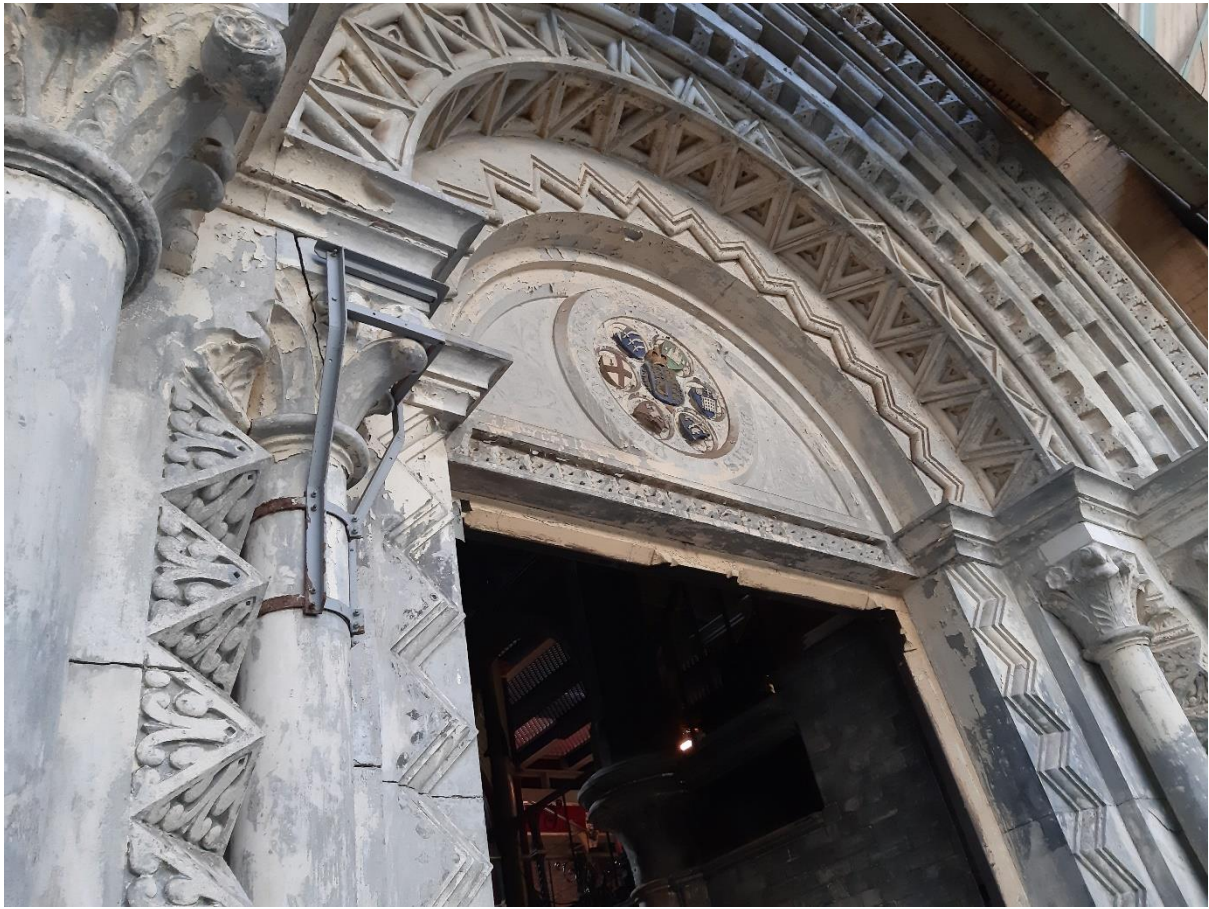
Original Front Door
